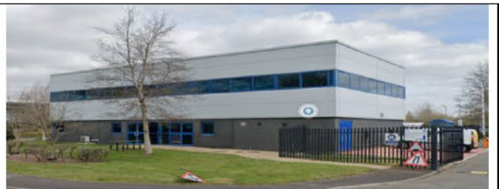
2 storey office Block
