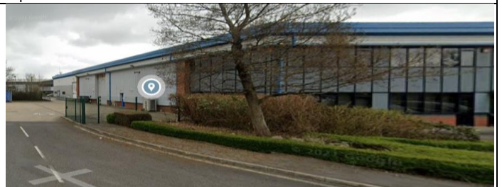
Industrial Warehouse/logistics Depot
