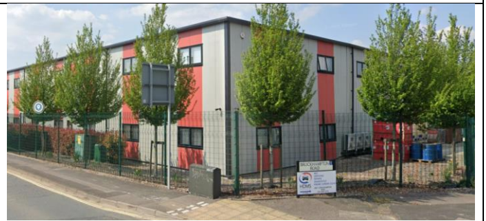
Warehouse with ancillary office – Built in 2016
