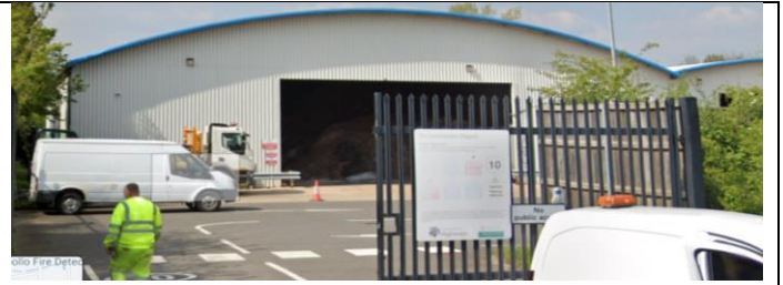
Large open Hangar – Grit storage
